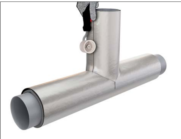
Figure 48: Securing overlap joints with seam roller
