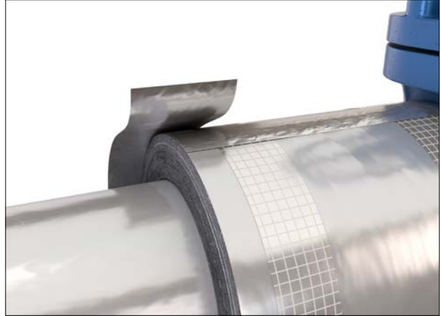
Figure 59: Application of vapour barrier tape (foil-faced butyl) at termination
