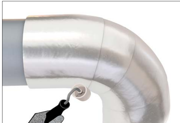
Figure 32: Securing overlaps down with seam roller
