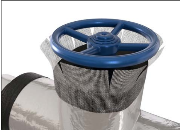
Figure 72: Application of the flexible reinforcing membrane at spindle insulation termination
