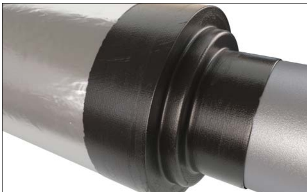
Figure 19: Application of vapour stop at insulation termination
