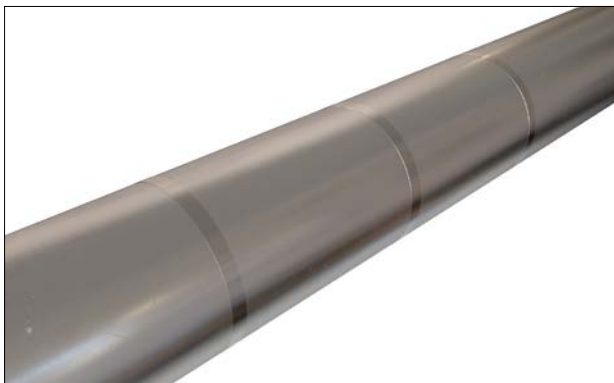
Figure 17: Apply cladding.
