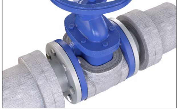
Figure 59: Packing out of air-space.
