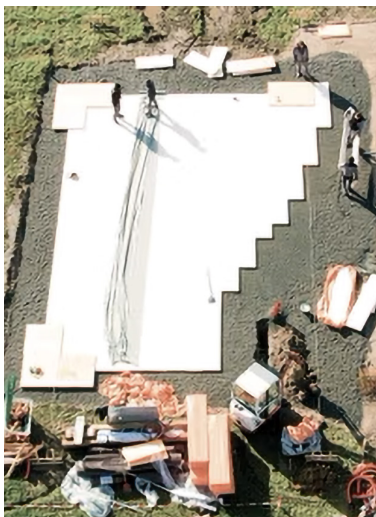
©Viebrockhaus: ArmaPET Eco50 perimeter and core insulation with a surrounding frost shield.
