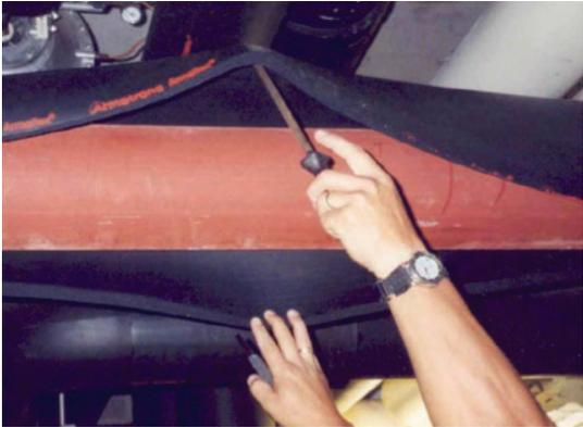
Figure 7: This cold water pipeline has been protected by Armaflex for 20 years - the picture shows maintenance inspection of the original system.
