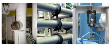
For a vibrating sound source - vibration isolate it from its supporting structure if that structure is likely to re-radiate the noise.
