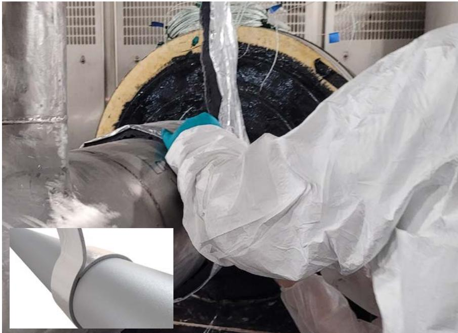
Figure 7: Measuring the diameter using material strips
