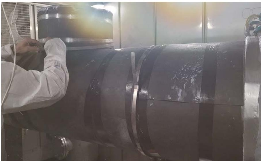
Figure 13: Installation of the Acoustic Barrier
