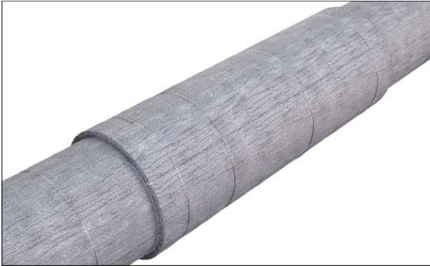
Figure 14: Securement of ArmaGel with stainless steel wires.
