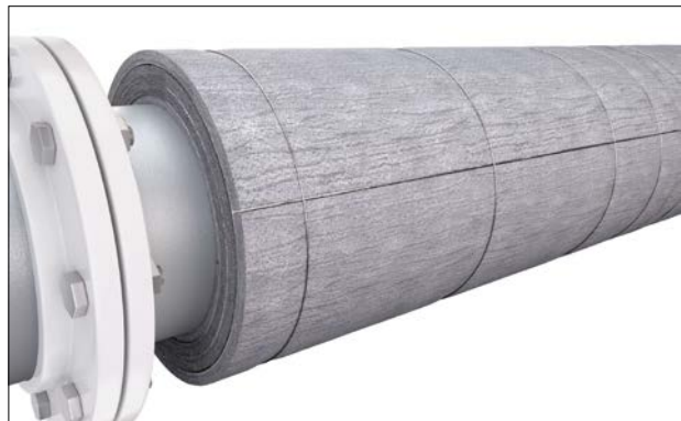
Figure 24: Positioning of final layer.
